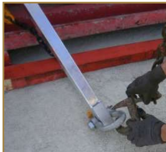
9 - Fix the crane slings onto the rings of the right and left brackets
